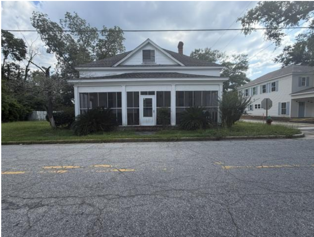
Subject property: View of the property from the ROW on West Inman Street, facing south.
