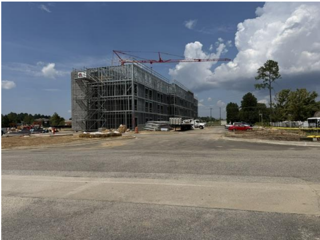
Subject property: View of the property from Stambuk Lane, facing north.
