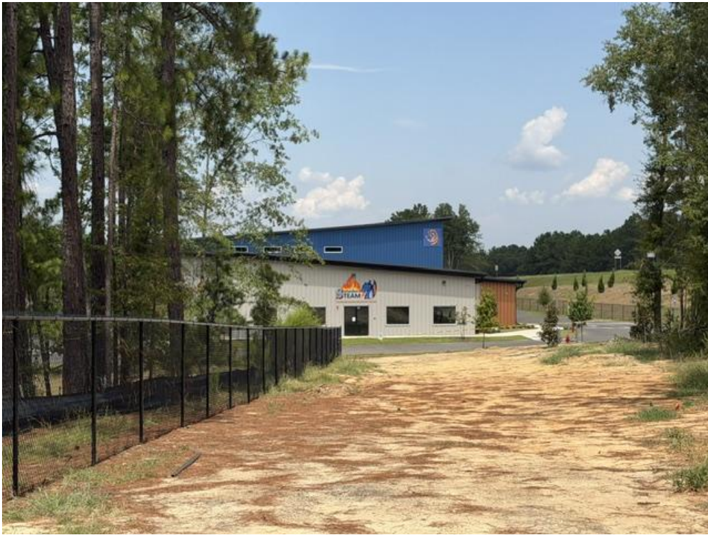
Subject property: view from the southwest corner from the ROW on East Main Street, facing north.
